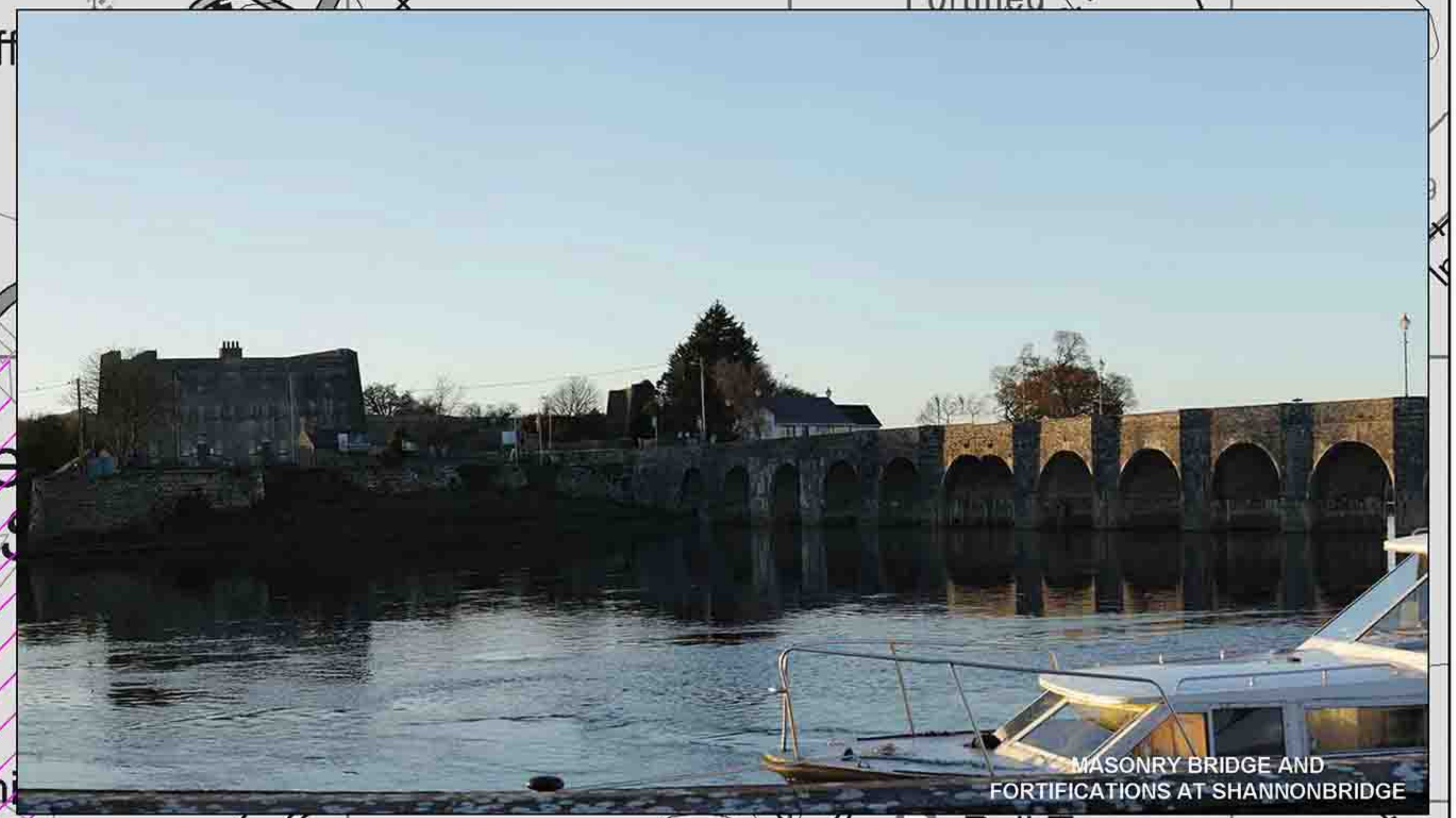
Masonry Bridge and Fortifications at Shannonbridge
